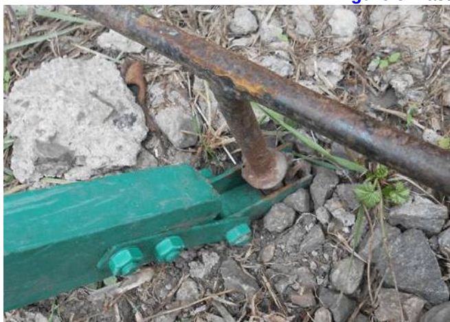
Figure 4 Strut fastened to the ground
