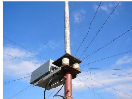
Ground Plane. Box with Matching Circuits
