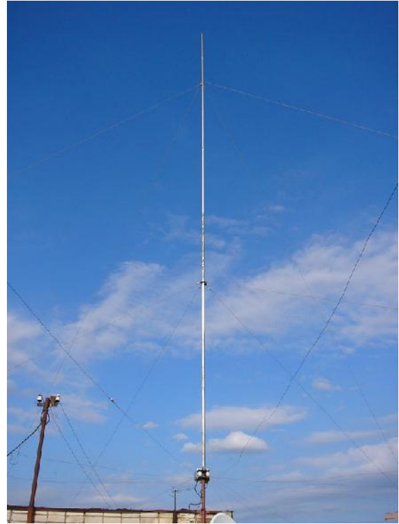
Ground Plane. General view
