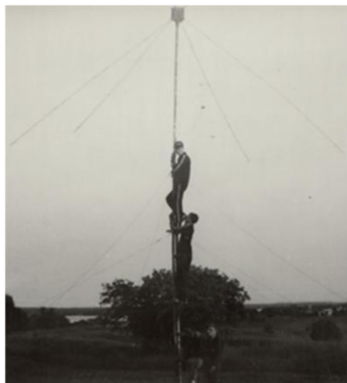
Installation of the Square for 10- 15- 20-meters
