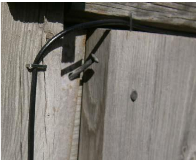
Figure 13 Stapled Wire of Beverage Antenna
